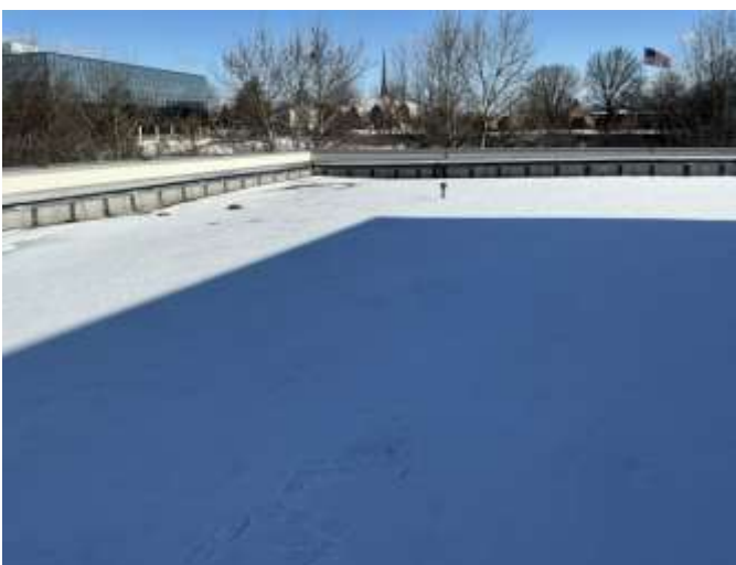
5 - PRIMARY ROOF OVERVIEW
