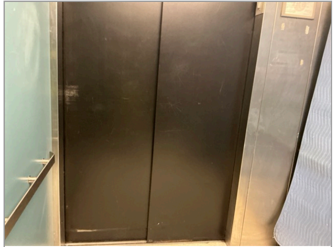
LOBBY LOOKING AT CABS (WITH DOORS OPEN)
