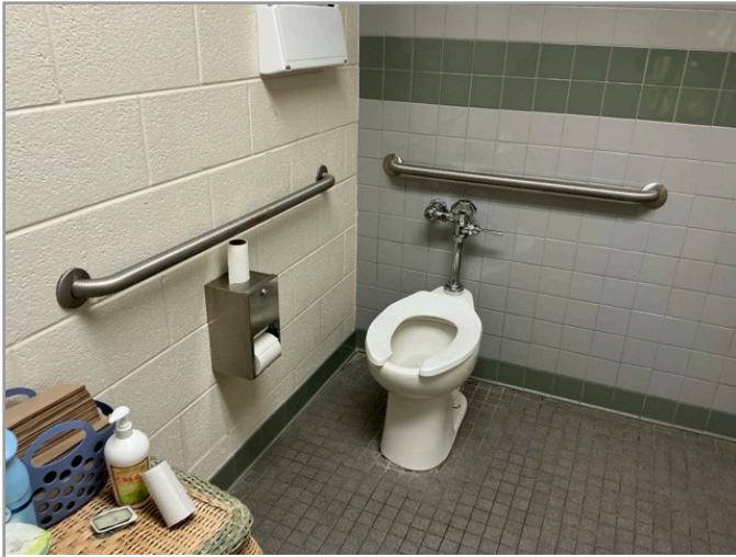
TOILET STALL OVERVIEW
